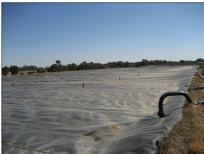
Figure 5.16 Example of a covered anaerobic lagoon installed at a rural pig production facility (Gopalan, 2013).
